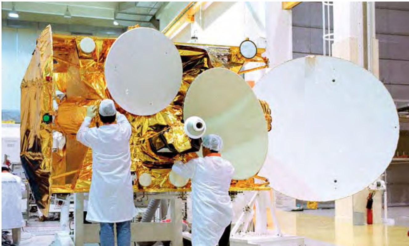
A satellite being integrated by Matra Marconi technicians EADS-Astrium
