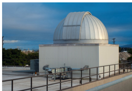
AeroTel sits on the roof of Aerospace's El Segundo, CA, lab facilities.
